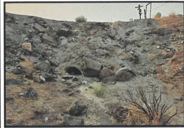
Existing 36" culverts. Upstream (northside) of Wayne Road
