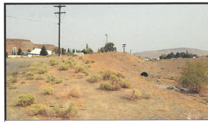
End of existing 72" CMP Culvert. Looking North.
